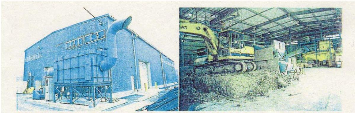
Fig. 2: The building, which adds additives to the soils carried in from the site (left). Inside, a plant, which mixes materials such as bark and chemical manures, was set up.
